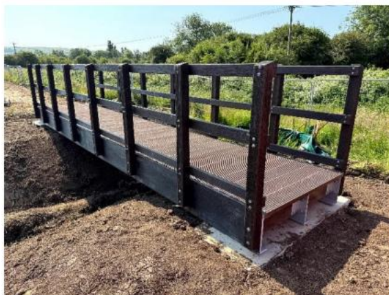
Image 2: Image shows complete installation of GPR footbridge 'Bridge 3'. Outstanding works is to only connect bridge to concrete foundations
