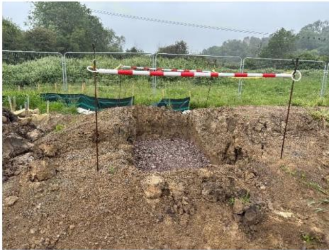
Image 2: Example of bridge foundation excavation.
