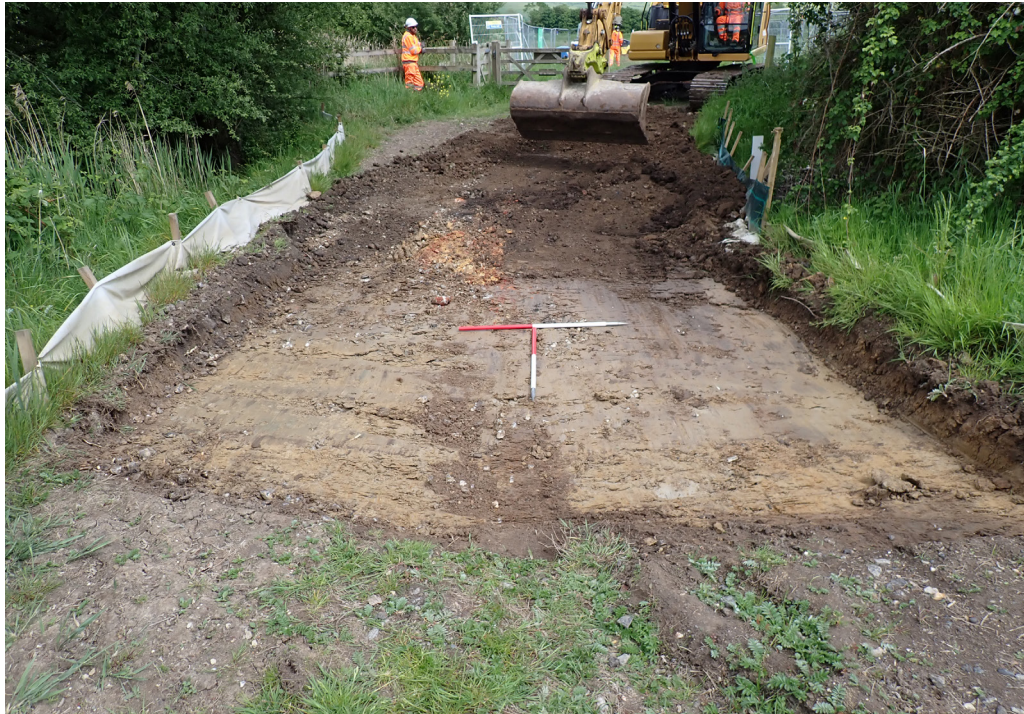
Fig. 3 Post ex shot for haulroad, East of brook
