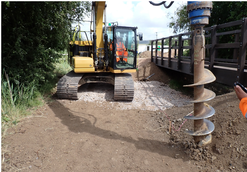
Fig. 6 Working shot of post hole being excavated
