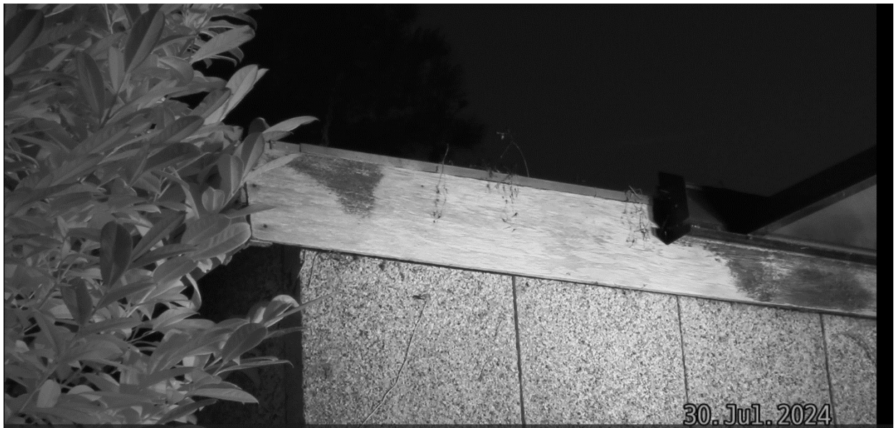
View from Canon XA11 infrared camera at survey position 3.
