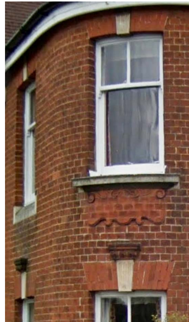
Decorative moulded brickwork and voussoir lintels with secondary tone for keystone bricks
