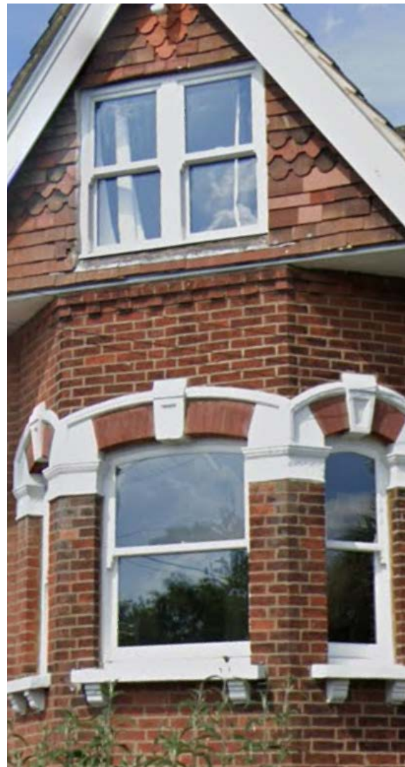
Sawtooth cornice and soldier course lintels
