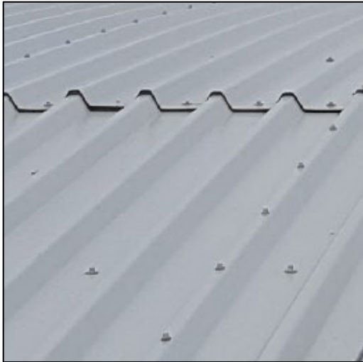
ROOF: LIGHT GREY PROFILED METAL PANELS
