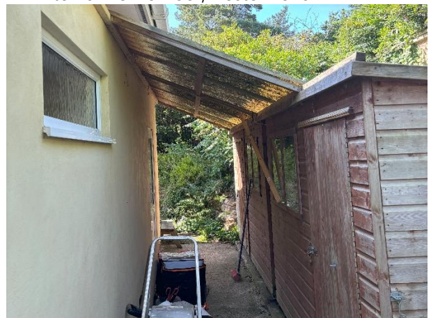
OB1: flat roofed shed adjacent to western side of B1.
