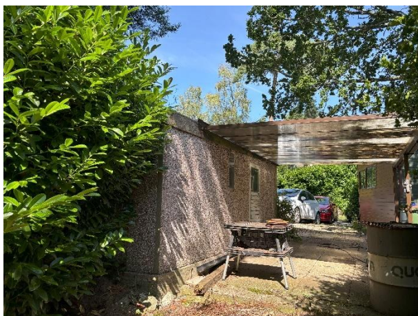
OB2: flat roofed garage north-east of B1.
