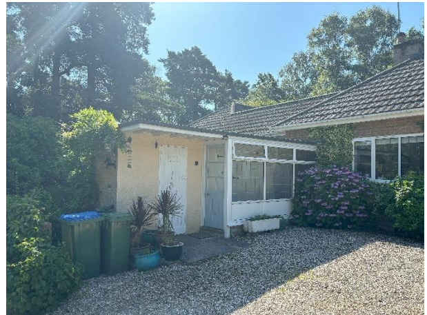
B1 (main house) northern aspect showing porch flat roof extension.
