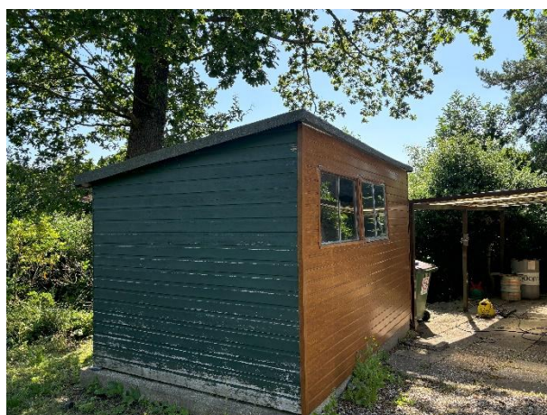
OB3: flat roofed shed north-east east of building OB2.
