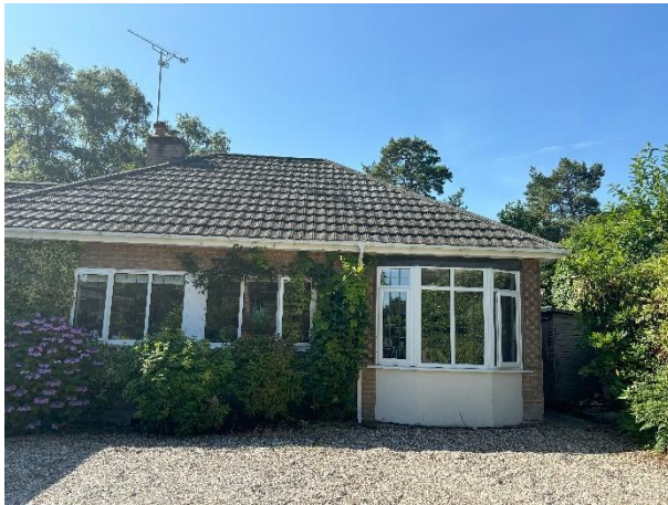
B1 (main house) northern aspect.
