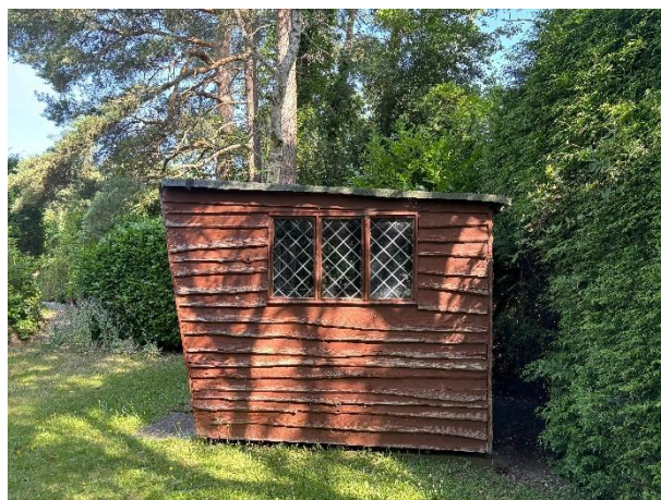
OB4: flat roofed shed east of building B1.
