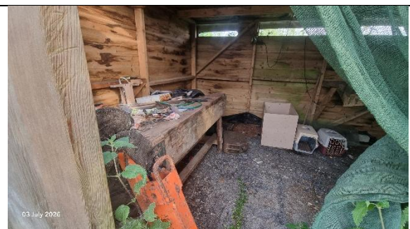
Plate 8. Inside of workshop (TN4)
