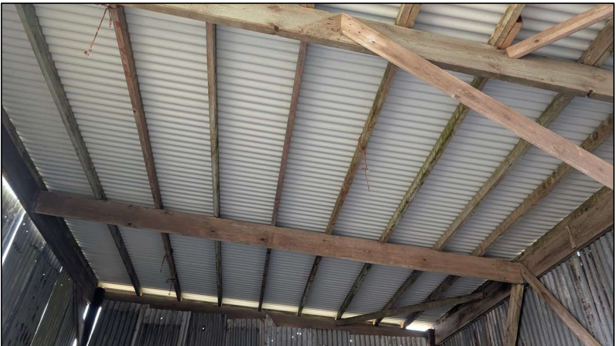
Photo 8 – Internal view of B2
