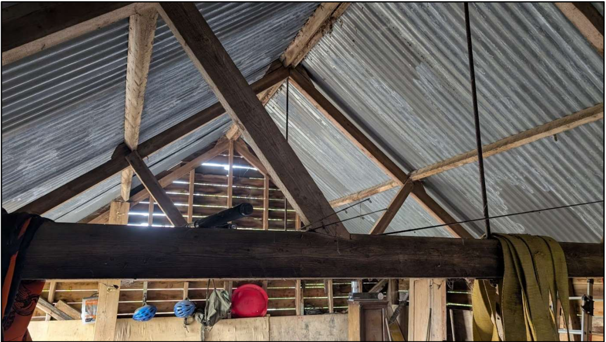
Photo 7 – Internal view of B1
