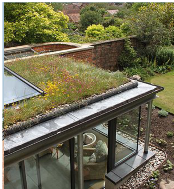
ROOF - Bauder Intensive Green Roof
