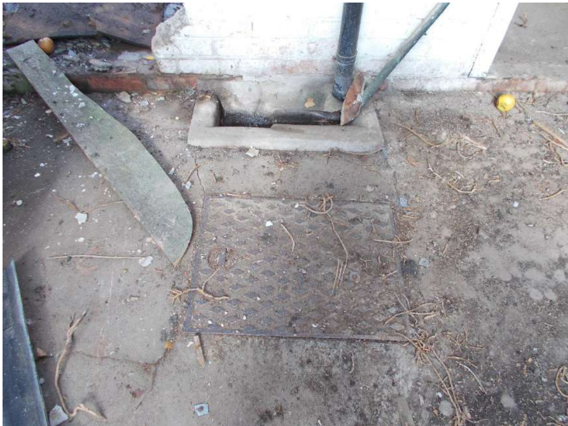
Drainpipe downpipes in garage
