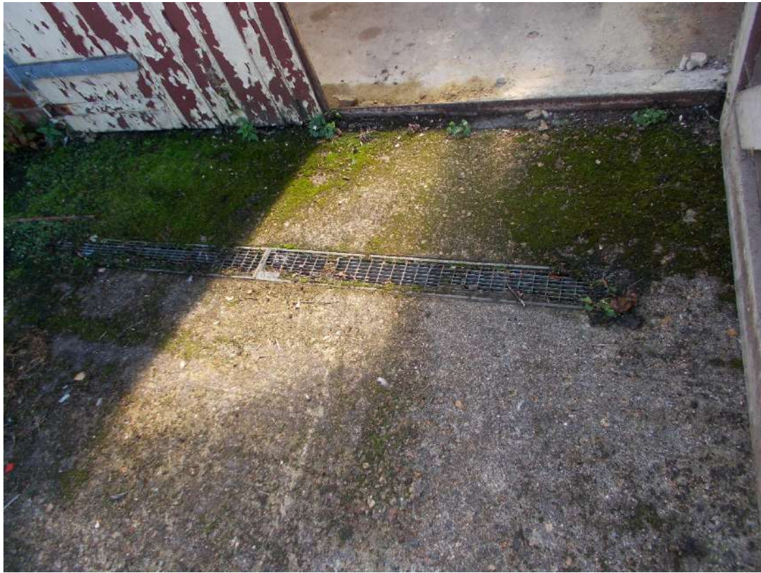
Strip drain in front of garage
