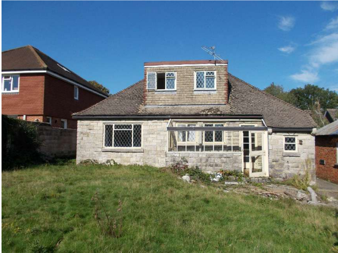
Rear of bungalow
