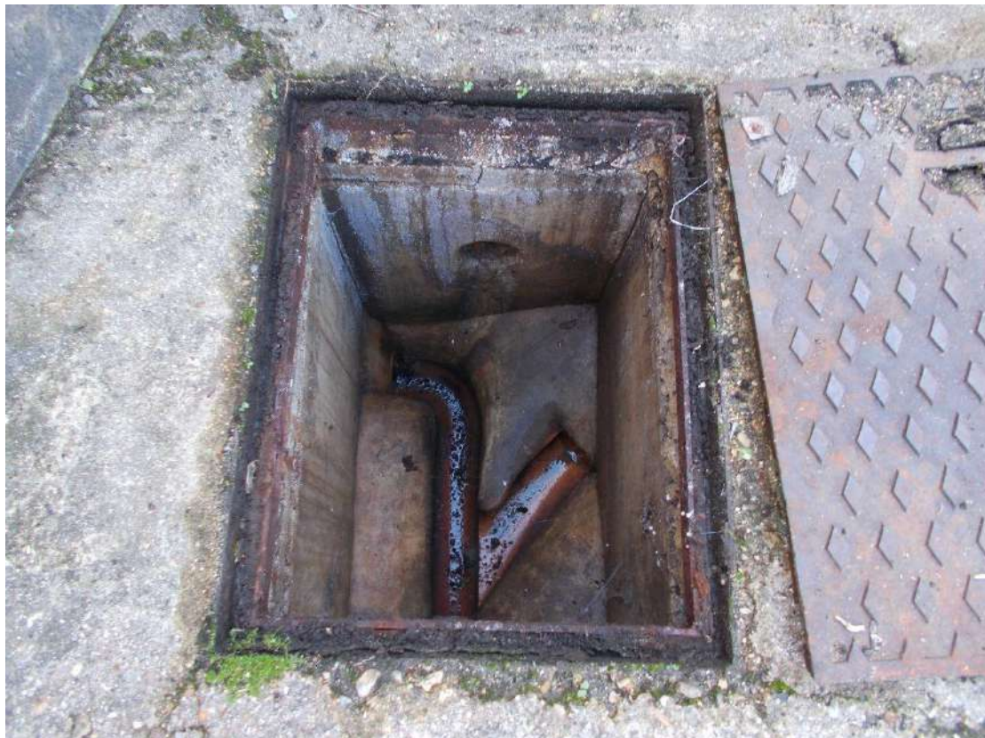
Existing drainage in front of house leading to public sewer
