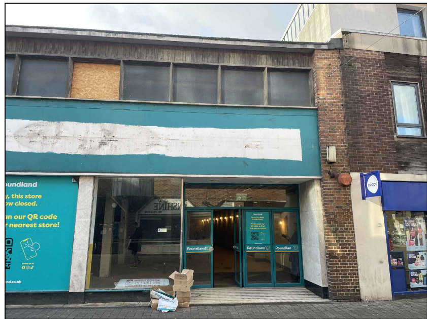
Photograph #2 Front Elevation - RHS
