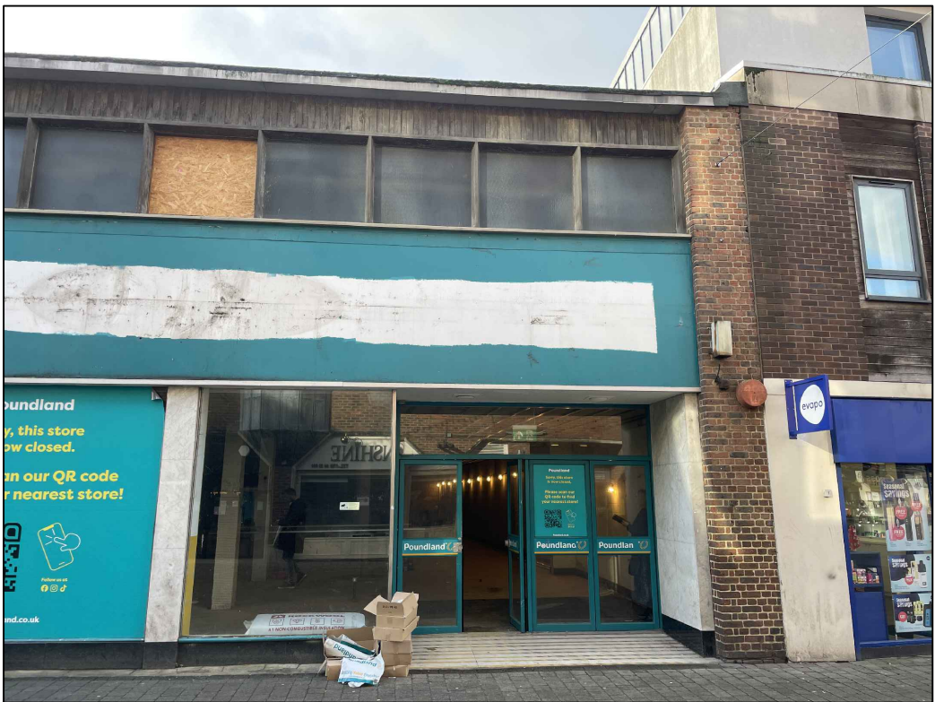
Photograph #2 Existing Front Elevation - RHS
