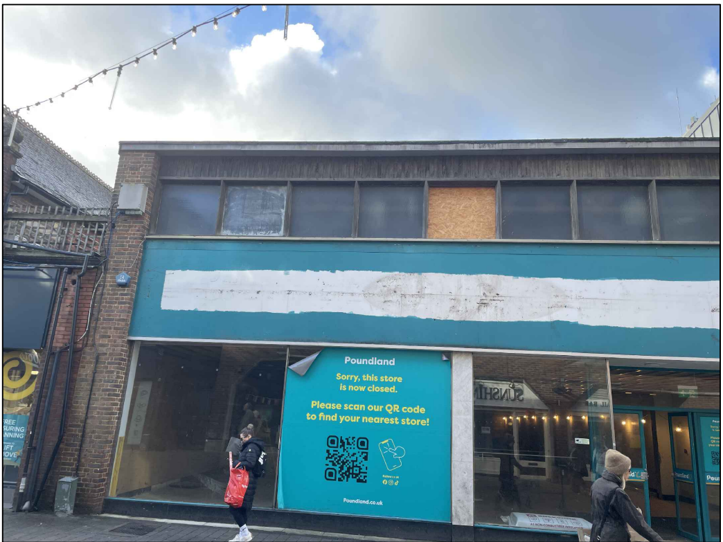
Photograph #1 Existing Front Elevation - LHS
