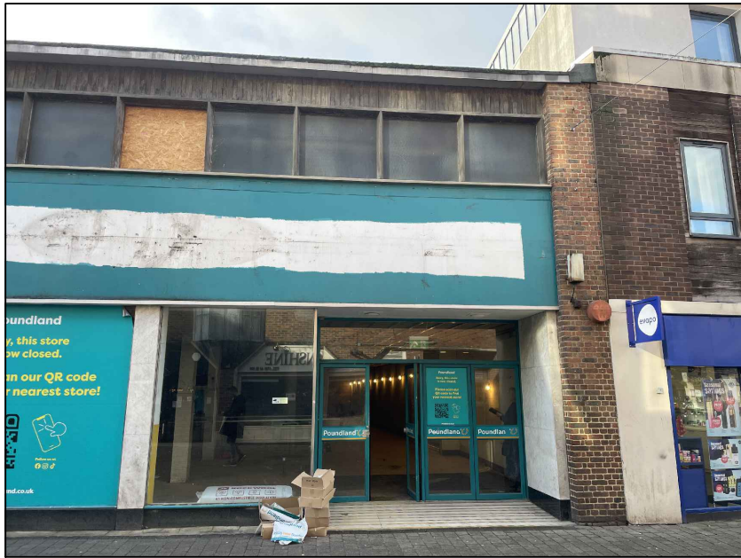
Photograph #2 Front Elevation - RHS
