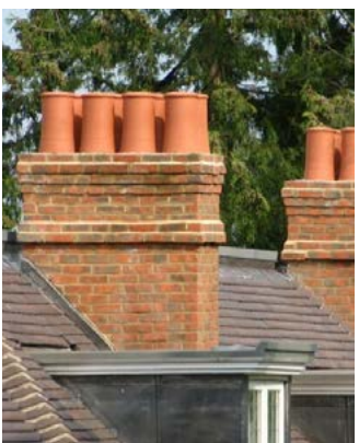
Sussex Stack Chimney
