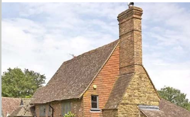
Gable and ‘Sussex Stack’ Chimney
