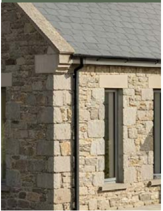
Stone Cornice and Quoin Detail
