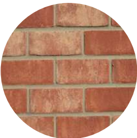
Light Red Brickwork
