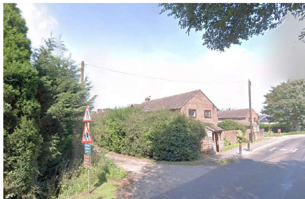
Fig 02. Street View of the Site Entrance on Storrington Road © Google Earth
