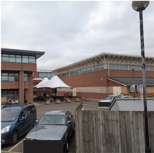
Existing bin store in the foreground, between the car park and the library. The proposals are to replace this with a landscaped area.
