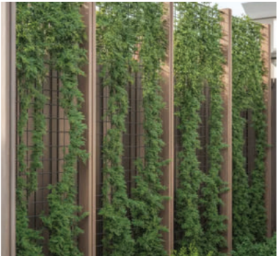
Screen planting to ASHP enclosure
