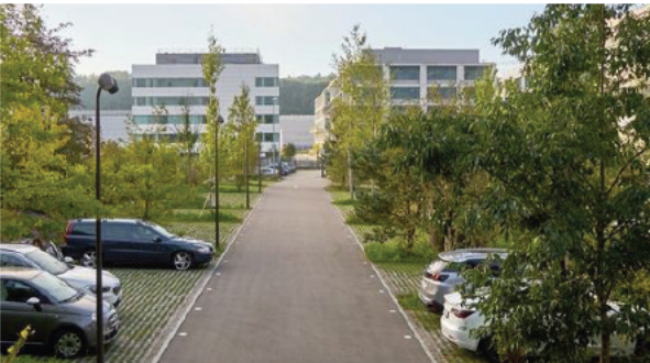
New car park arrangement with permeable paving in parking bays
