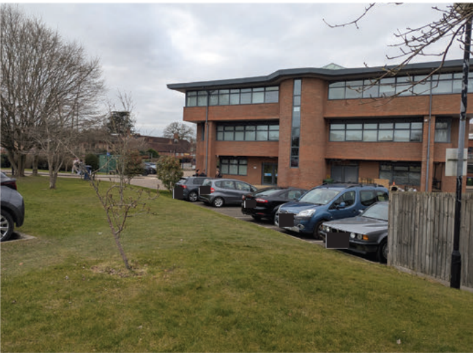
The southeast side of the Library. Bin store (right). Level change up to the car park.
