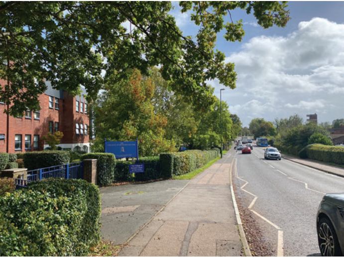
The Buckle Building (1976). Facing south on Hurst Road.
