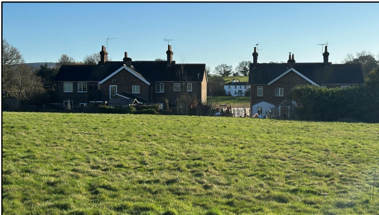
Photograph 3: View south across field to houses of the Henfield Conservation Area showing houses that have been flooded by surface run-off.
