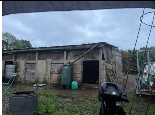
Photograph 9 – Surveyor position two by the southwest elevation of the survey building. Image of view at the start of the survey on 5 th June 2025.
