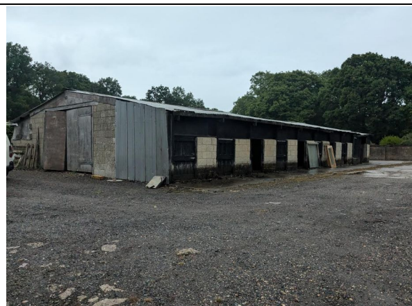
Photograph 11 – Surveyor position three by the south and east elevations of the survey building. Image of view at the start of the survey on 5 th June 2025.
