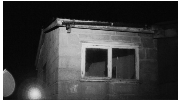
Photograph 14 – Surveyor position four, camera image of view at dark on 5 th June 2025.
