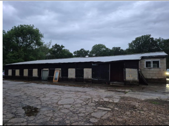
Photograph 7 – Surveyor position one by the east elevation of the barn building. Image of view at the start of the survey on 5 th June 2025.
