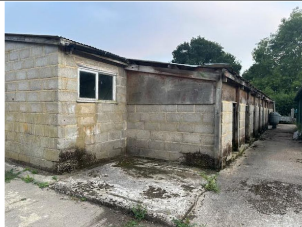
Photograph 15 – Surveyor position one by the corner of the north and west elevation of the survey building. Image of view at the start of the survey on 23 rd July 2025.
