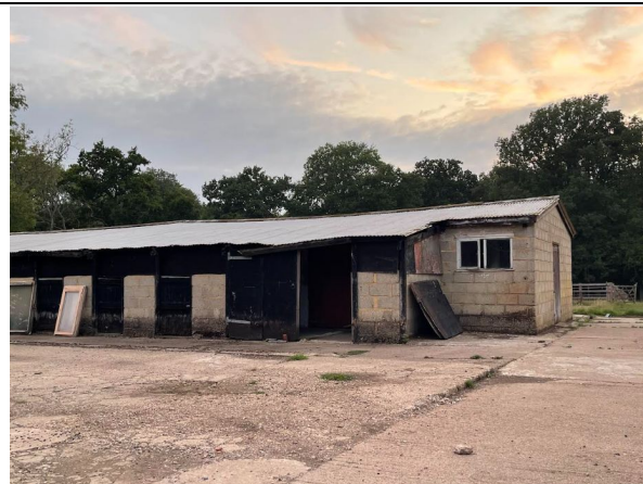
Photograph 17 – Surveyor position two by the corner of the north and east elevation of the survey building. Image of view at the start of the survey on 23 rd July 2025.
