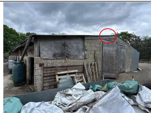
Photograph 23 – The location of the likely pipistrelle emergence on the first survey on 7 th May 2025.
