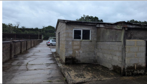
Photograph 13 – Surveyor position four by the corner of the north elevation of the survey building. Image of view at the start of the survey on 5 th June 2025.
