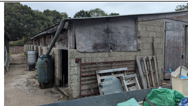
Photograph 21 – Surveyor position two by the south elevation of the survey building. Image of view at the start of the survey on 7 th August 2025.
