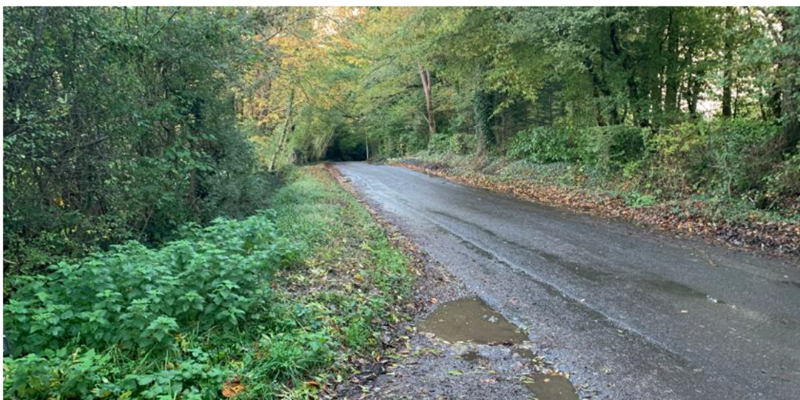
Photo 26: View to the North (Left) on Exit
