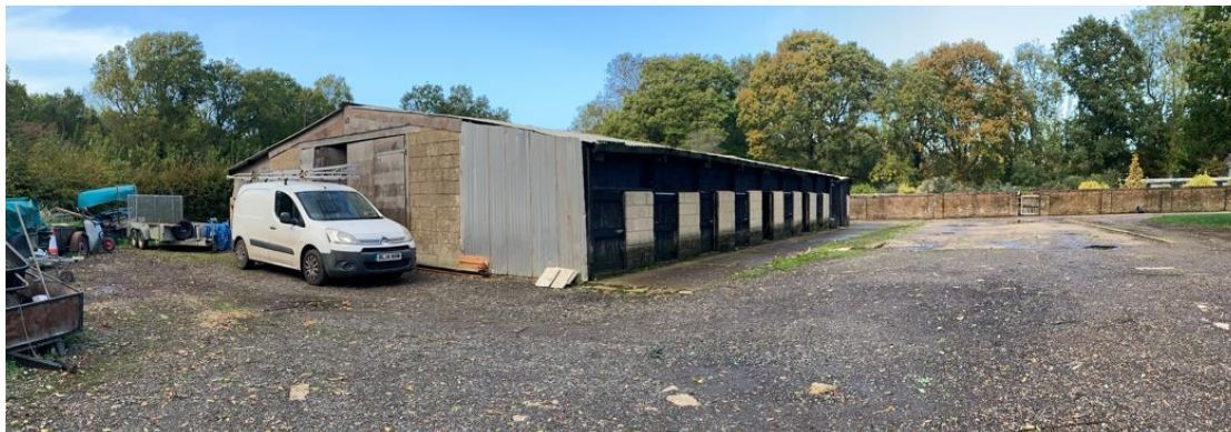
Photo 10: The Building from the South
