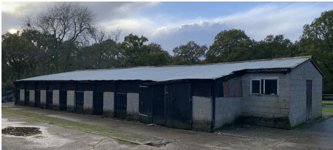
Photo 3: The Application Building
