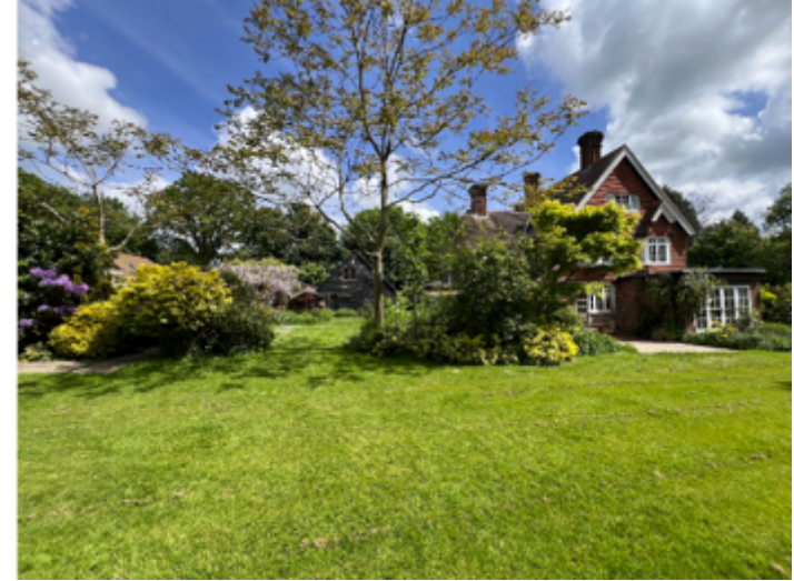
Figure 6 - view of dwelling from south
