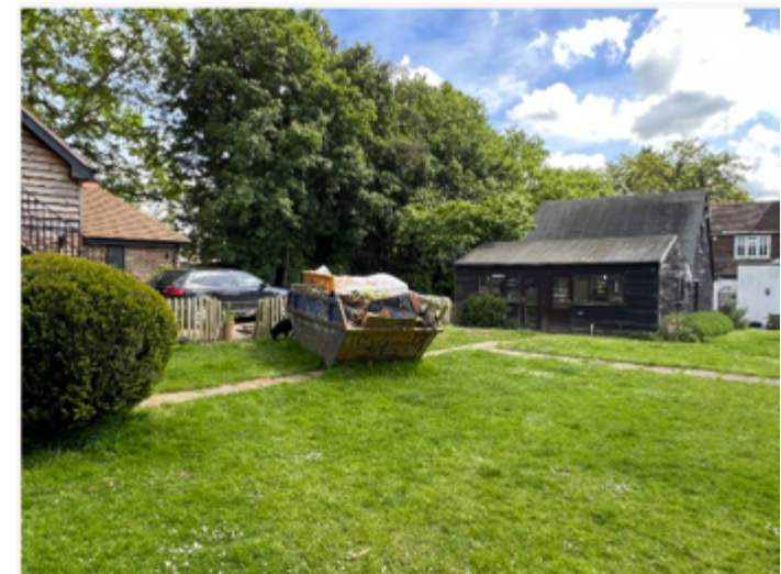
Figure 11 - Existing annexe and garage
