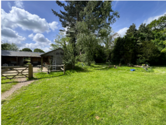
Figure 9 - Existing stable building
