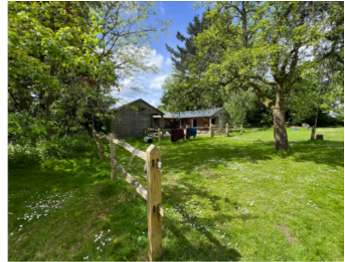
Figure 7 - existing stable building
