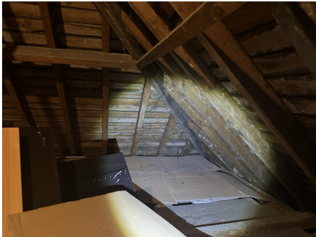
Internal void of B1
