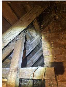
Internal void of B1
