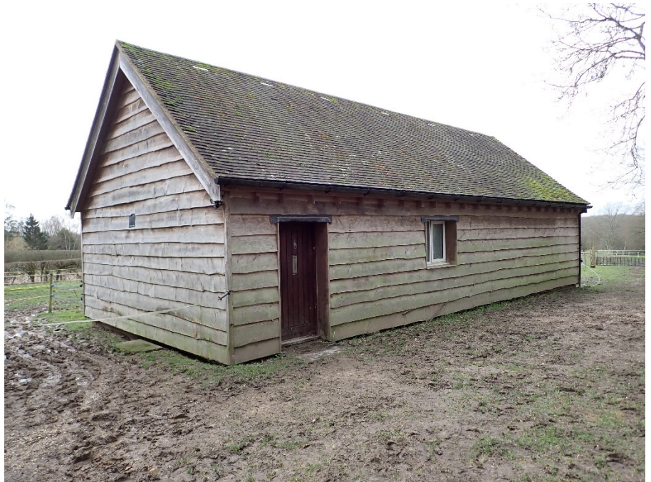
2.1 Existing Stable Barn, showing east & north elevations
