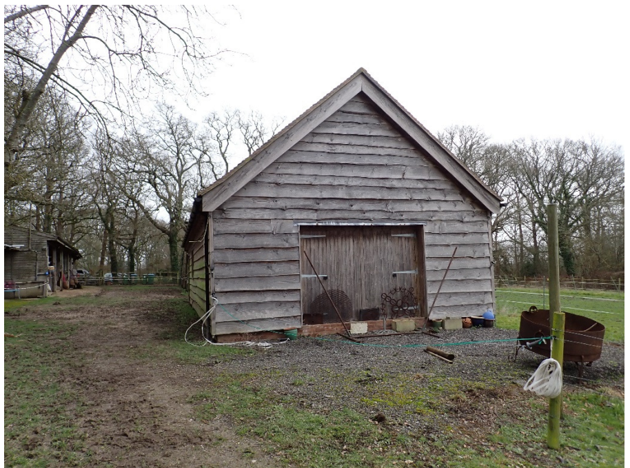
2.2 Existing Stable Barn, showing west elevation
