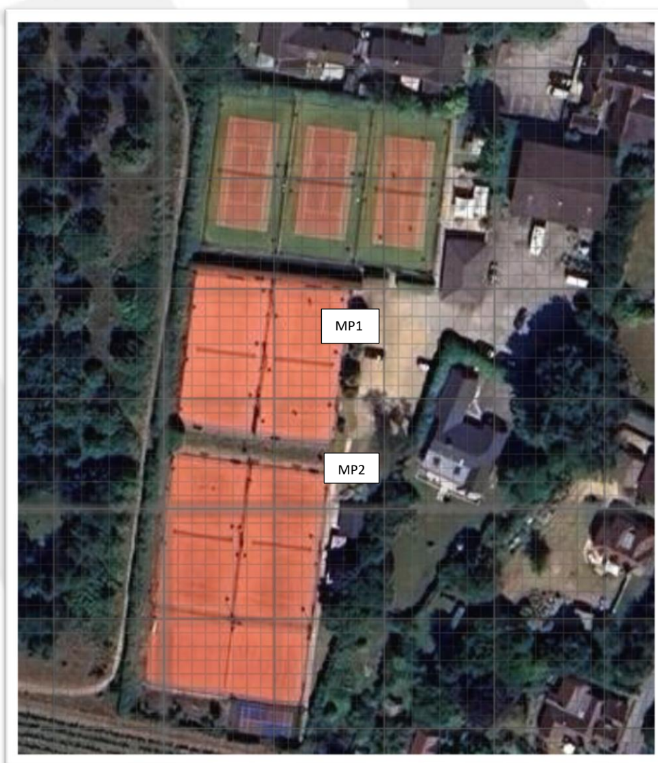
Fig 5.1 shows the location of measuring points at the Site
