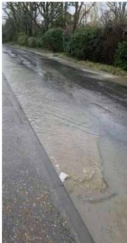
Chapel Road – Looking towards Proposed Site Entrance
