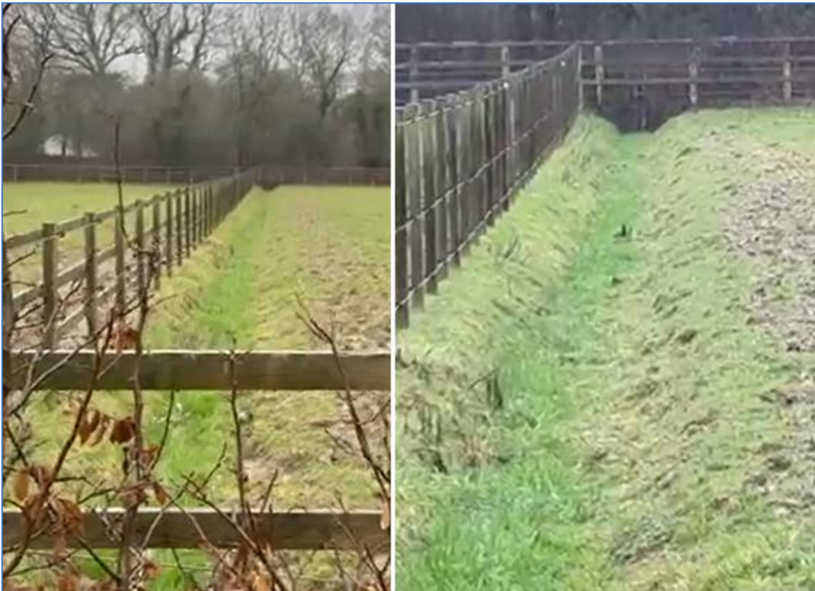
Figure 6: Photos of the Drainage Ditch on Site (Source: Equine America UK)
