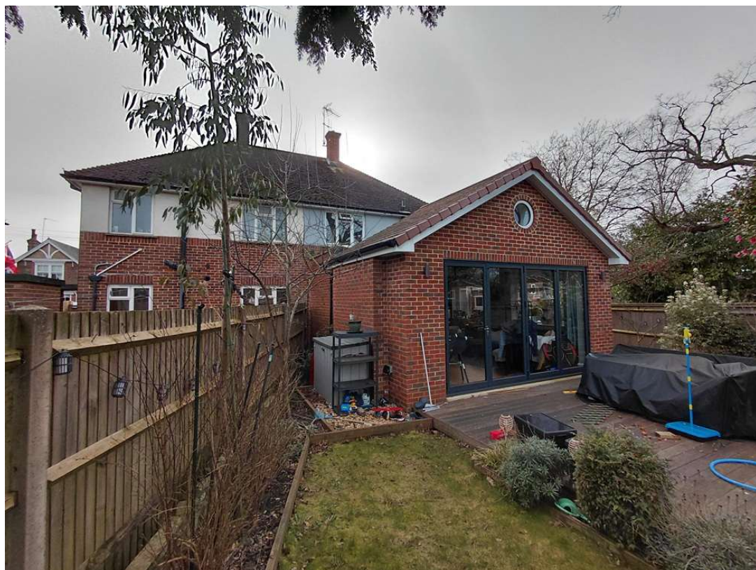
Rear Of Subject Site- No. 25- Above
