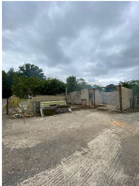
Photograph B : The garage during demolition
