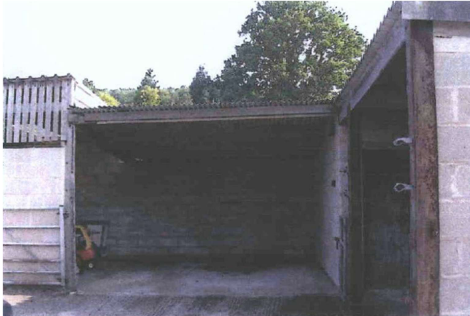
Photograph A : The Garage prior to demolition
