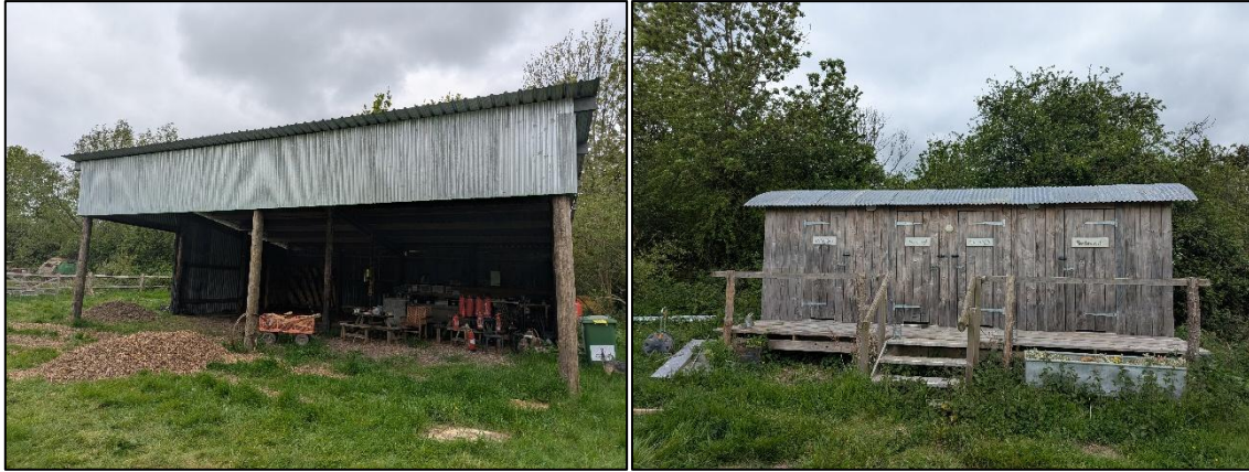
Photographs of seating area (left) and toilet and shower facilities (right)
