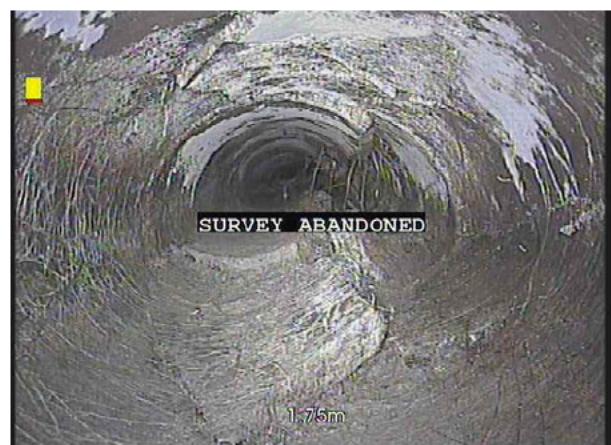
6, 00:00:57, 1.75 m Survey abandoned, Unable to pass - assumed redundant
