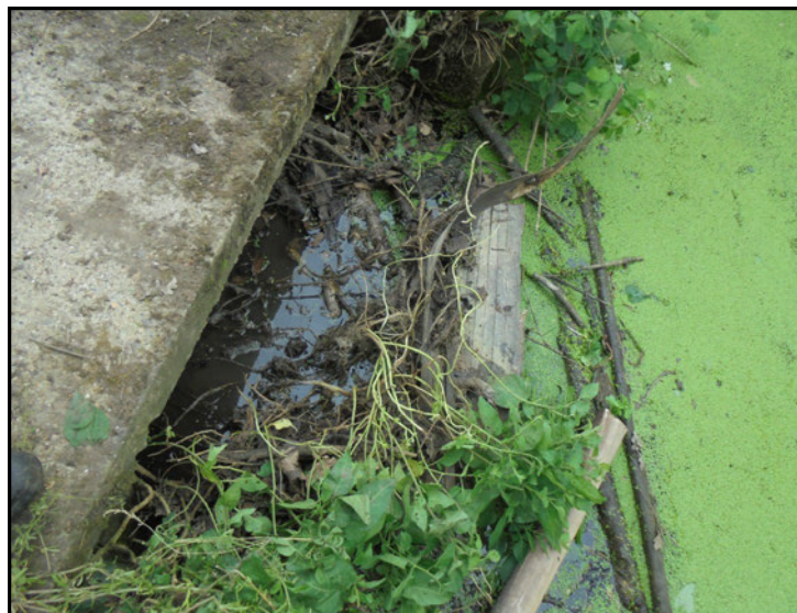
OF2 INTO SLABBED CHAMBER
