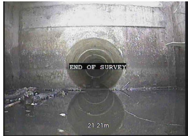
2, 00:01:43, 21.21 m Finish node, manhole, reference: IC1
