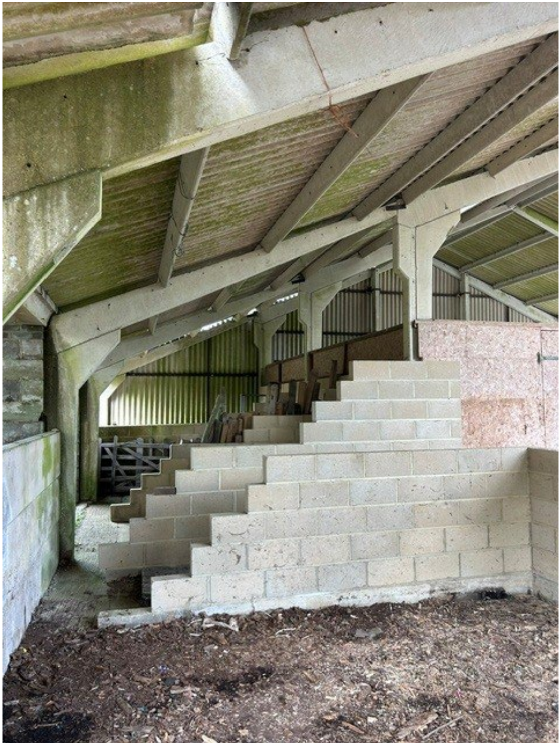
1Internal view of low separating walls
