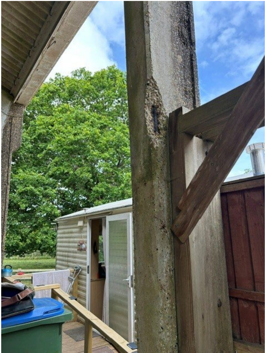
Figure 3 Column next to Mobile home
