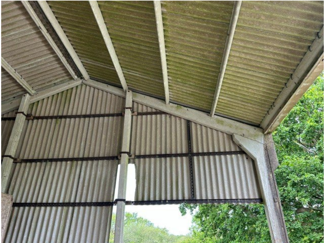
Internal rear elevation
