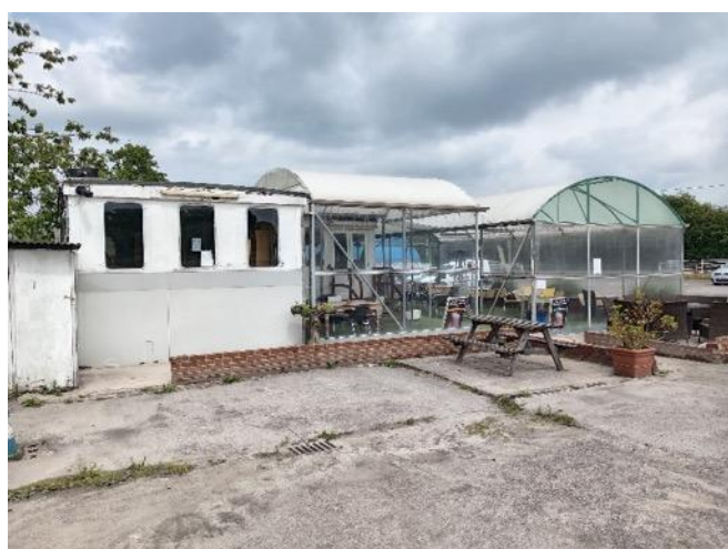
Photograph 7. B7 NHP Allocation café and car wash facility
