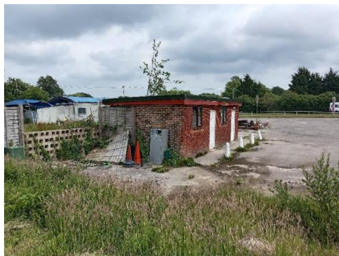
Photograph 6. B7 NHP Allocation toilet block
