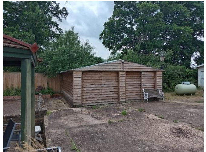
Photograph 4. B2 wooden garage northwest of B1.
