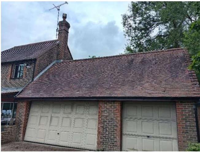
Photograph 3. B1 attached garage with loft void over
