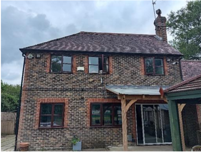
Photograph 1. Northwest elevation of B1, garage to right of photograph
