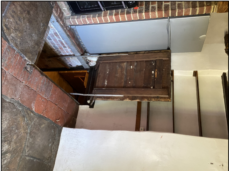
Access hatch in kitchen
