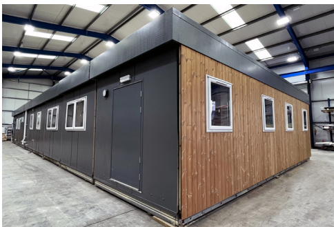
Figure 2. Diagrammatic representation of an 8-bay modular building
