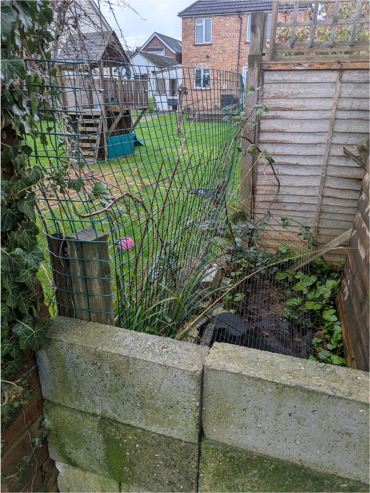
Existing gap in boundary fence – new fence to include small mammal access
