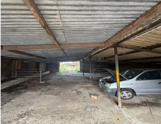
Plate 11: Corrugated Roofing in Barn
