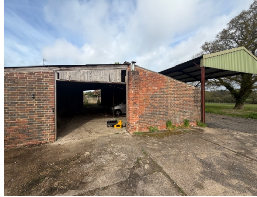
Plate 12: Single Layered Brick Frontage
