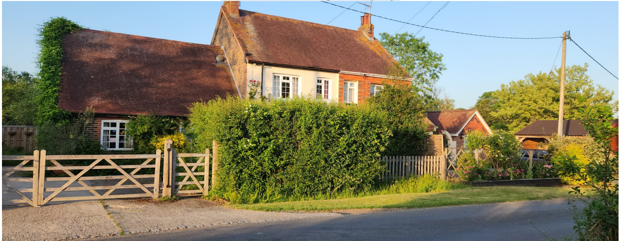
Photo 1. Front elevation, Street scene showing 1 and 2 Oakwood Cottages from the road.
