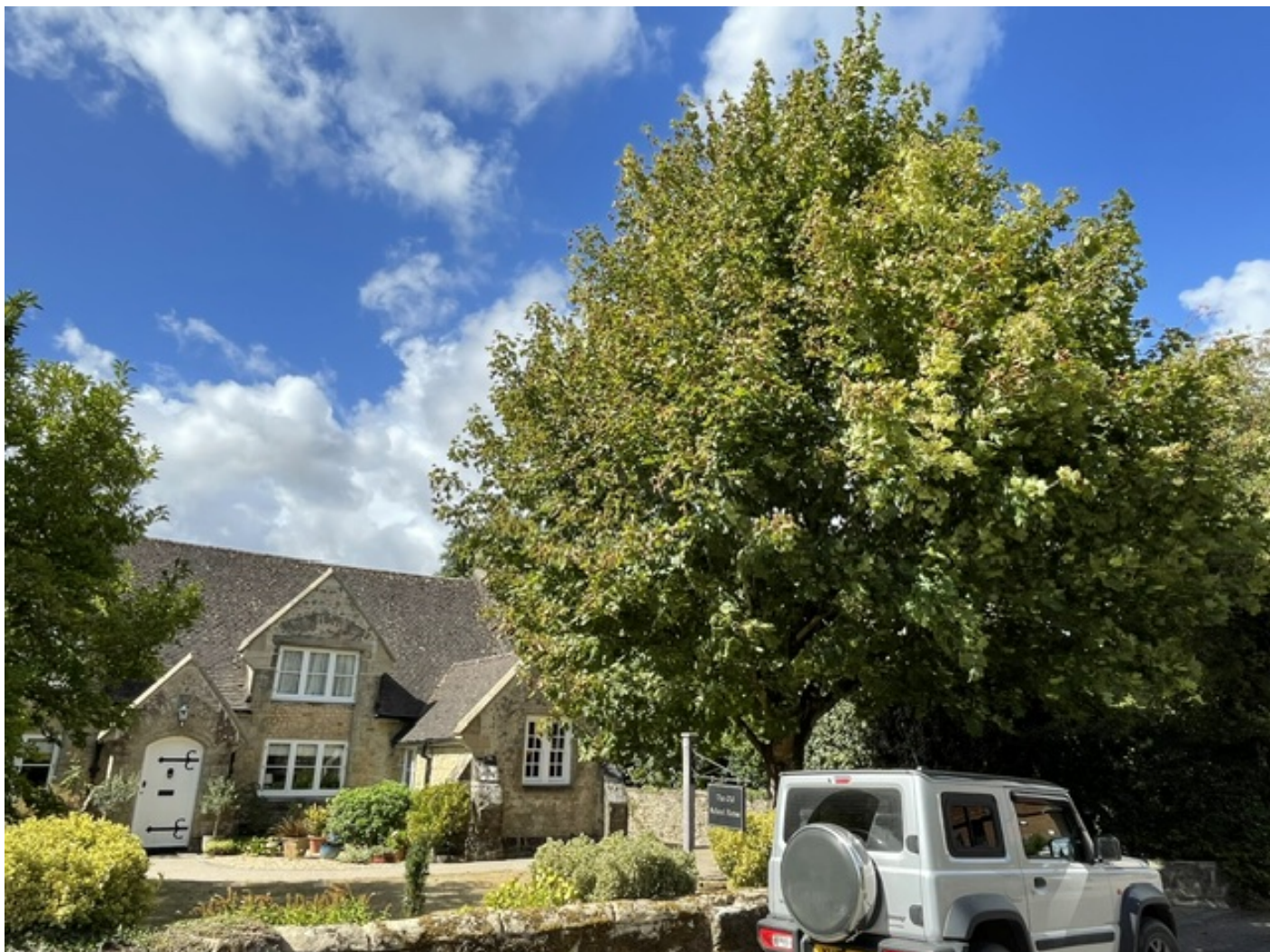
View from the street looking onto Old School
