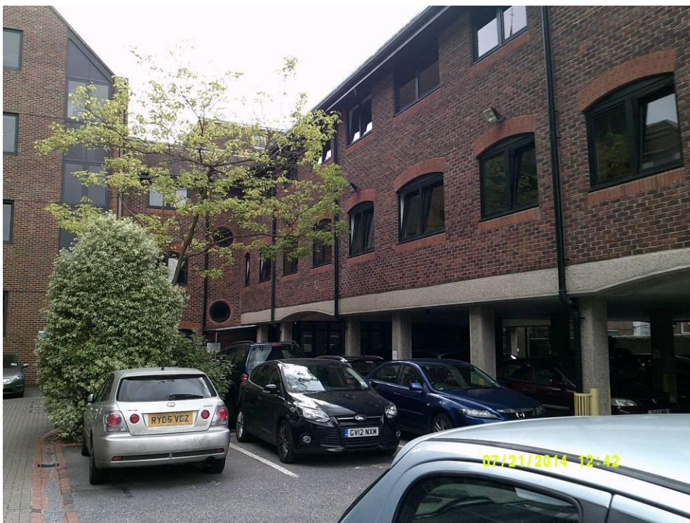
Plate 4: View south of western boundary wall and car park
