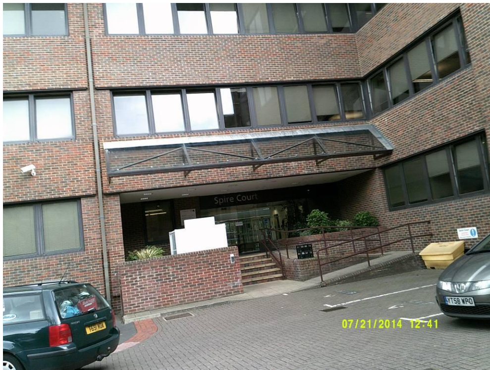
Plate 2: View west of car park
