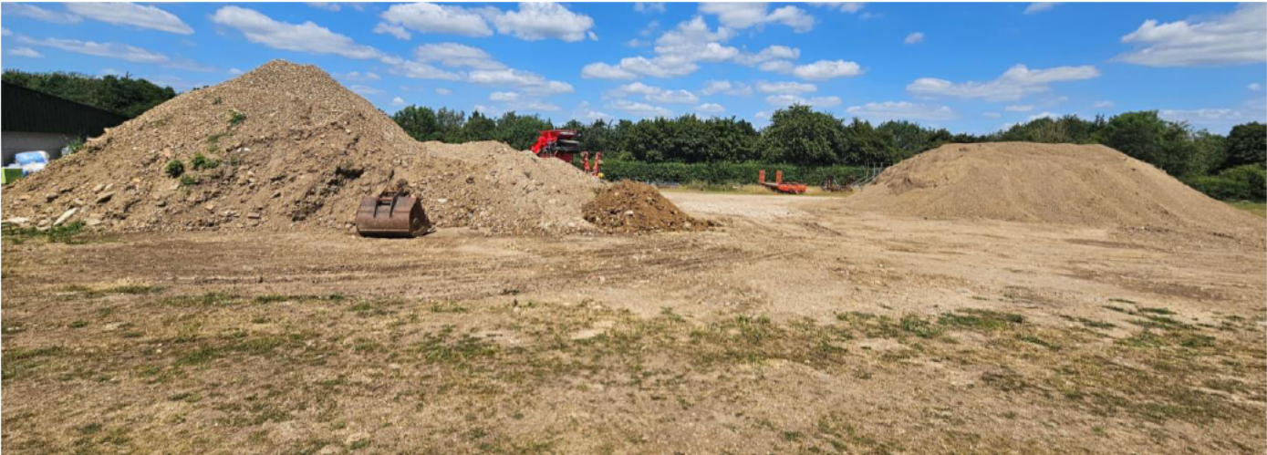
Photo 2: Displaying areas of modified grassland of poor condition surrounding the scrap material heaps south of site.
