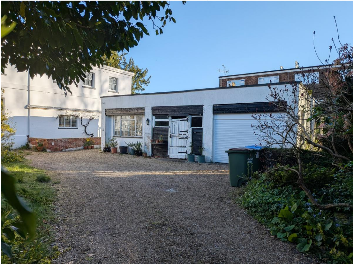
Existing garage building and workshop
