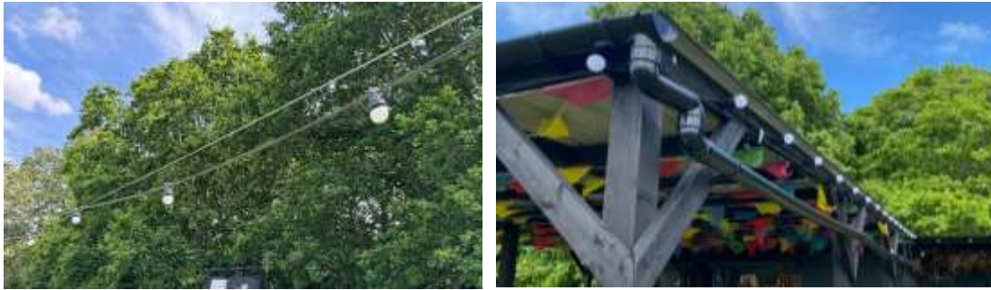
Photograph 1 & 2. Lighting at the Site
