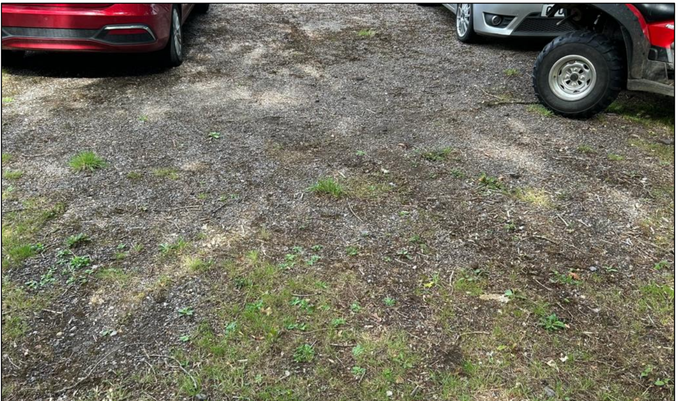
Photograph 2. The surfacing of the existing car parking area.
