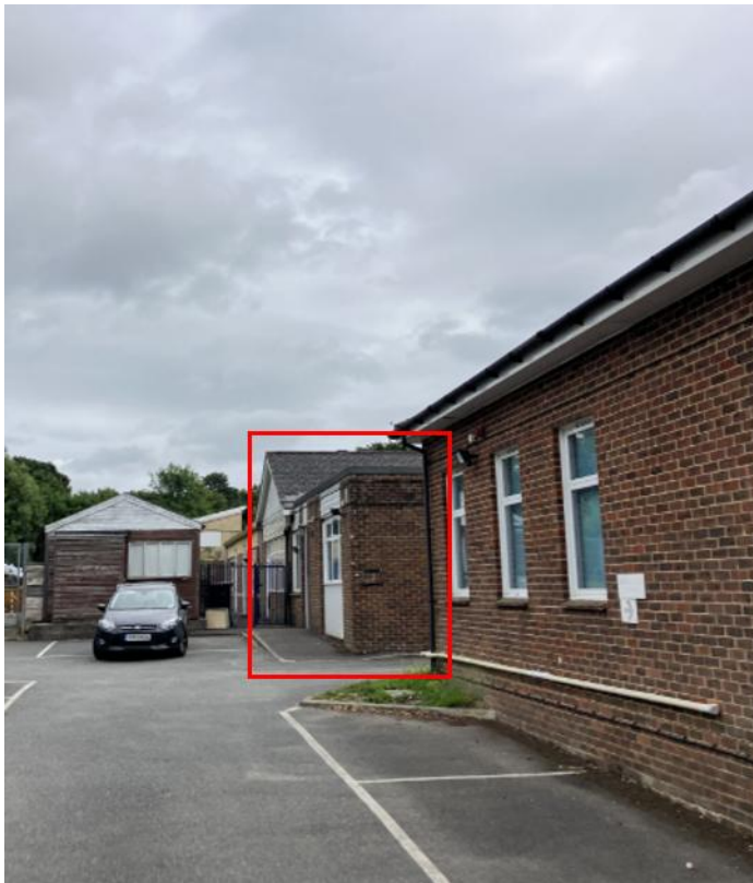
St Mary's C of E Primary School: View of building with flat roof proposed to be used to install one of the south facing arrays (highlighted)
