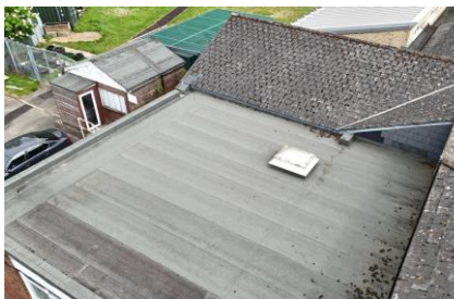
Flat roof building view looking east
