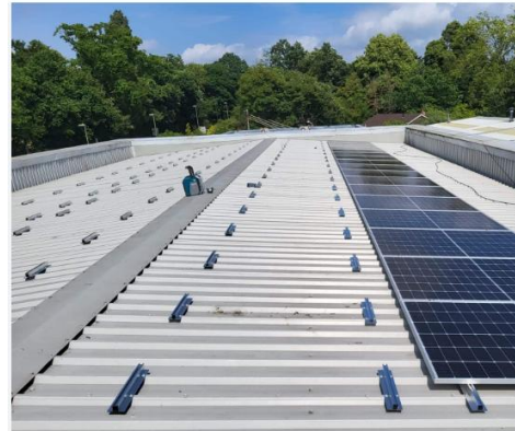
Rail mounting system standing seam
