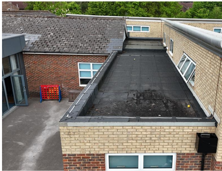
Pitched roof building adjacent flat roof view looking north
