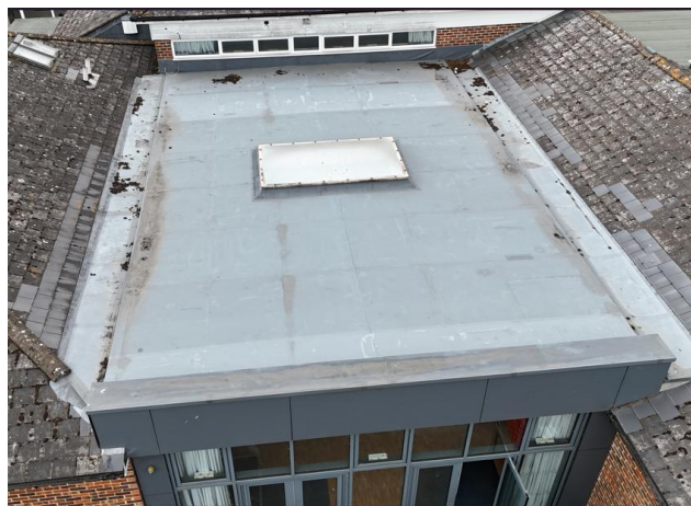
Pitched roof building view looking north
