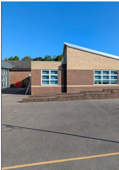
Pitched roof building view looking north
