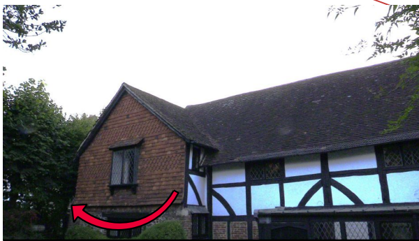
Photograph 1. Emergence of a common pipistrelle or soprano pipistrelle from behind a hanging tile on the southeast corner of the property at 32 minutes after sunset during survey visit 1 (Roost 3).
