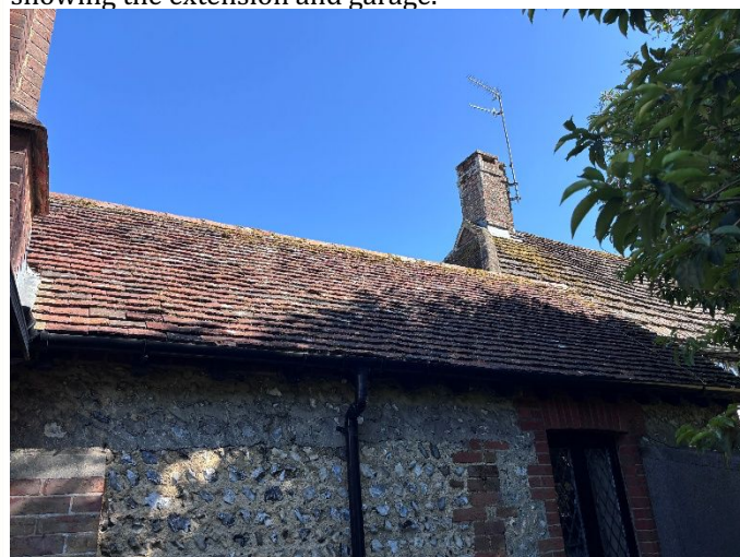
Photograph 5. Northern and western elevations of the property.
