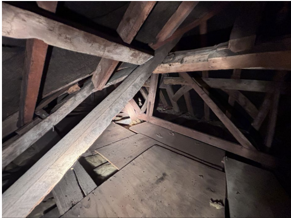
Photograph 1. Photograph of Roof void 1 taken from the southwest corner.
