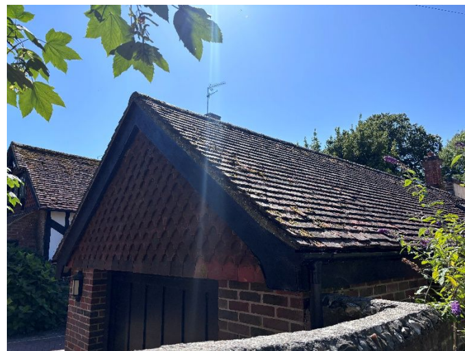
Photograph 4. Northern elevation of the garage.
