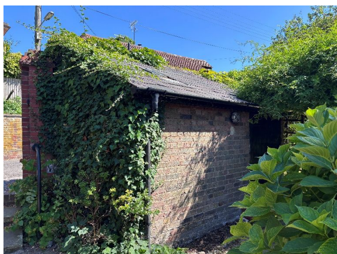
Photograph 6. Western elevation of the outbuilding.
