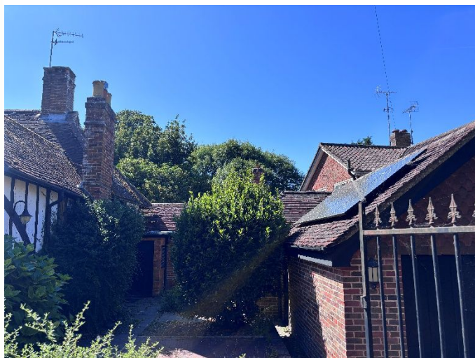
Photograph 3. Eastern elevation of the property, showing the extension and garage.
