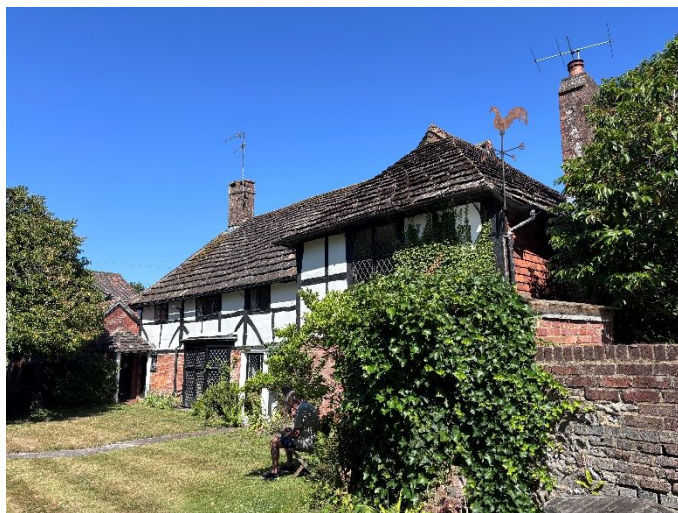
Photograph 1. Western and southern elevations of the property.
