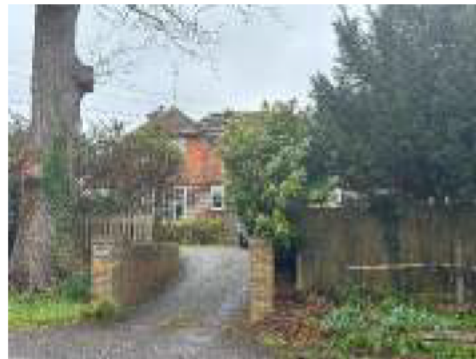
Properties in Henfield Road
