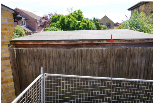
ADJACENT NEIGHBOUT FLAT ROOF OUTBUILDING
