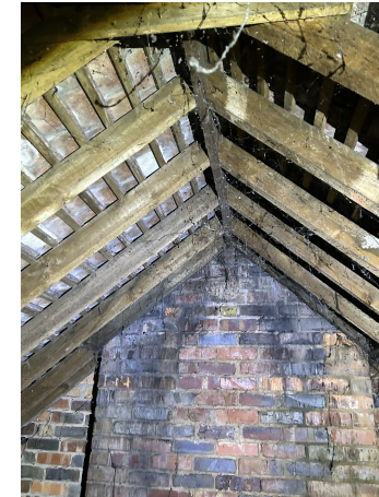
Figure 1a: B1 loft void.
