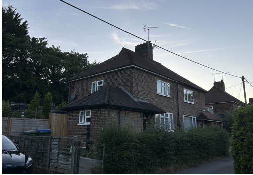
V1 B1-1 surveyor photo
