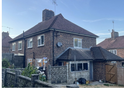
V1 B1-2 surveyor photo
